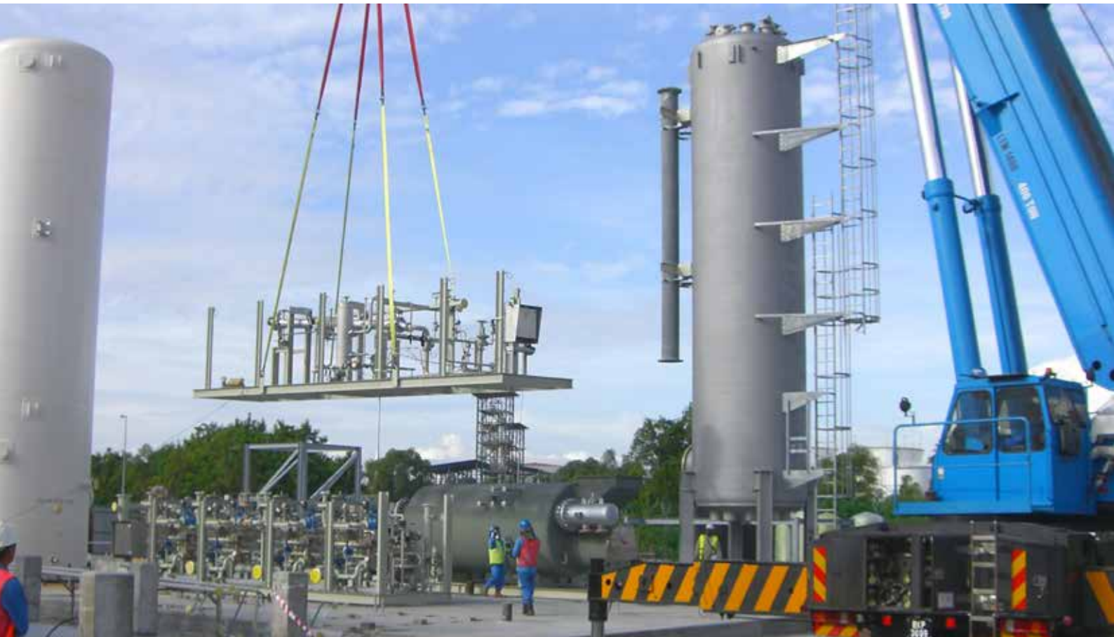
Natural gas steam reformer capacity 5000 Nm 3 /h during erection
