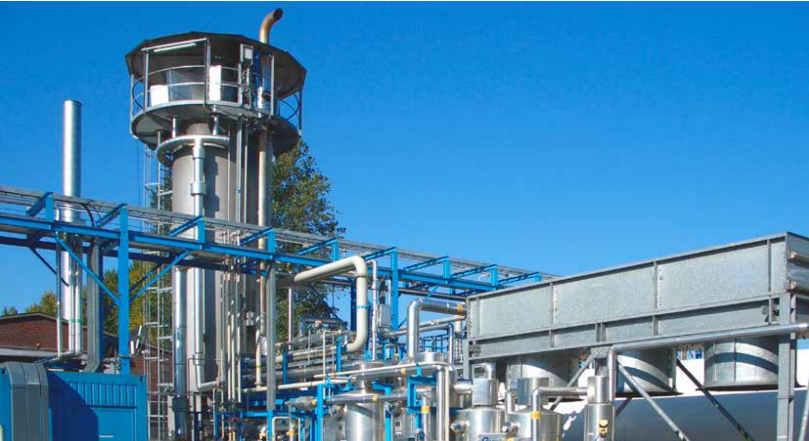
Syngas Plant for 1500 Nm 3 /h
