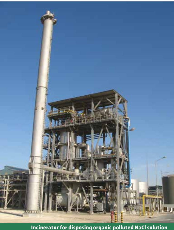
Incinerator for organically polluted NaCl solution
