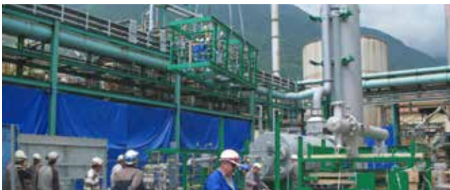
Placement of skid on prepared foundation
