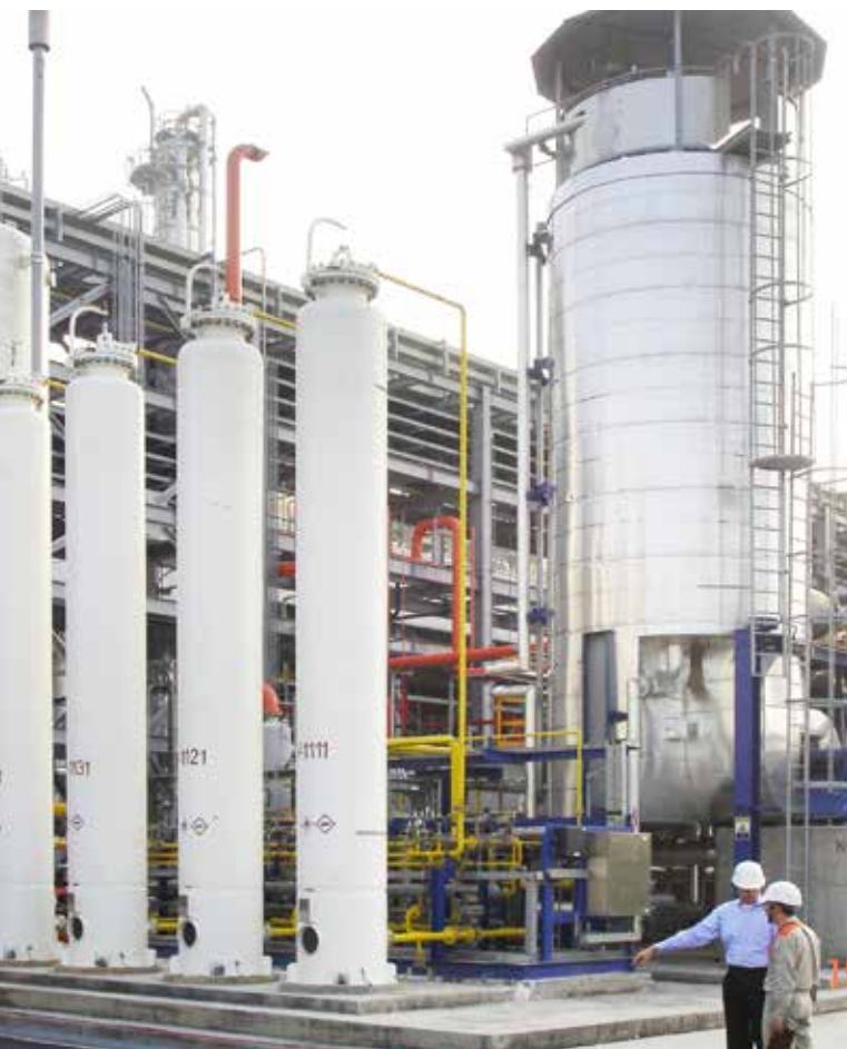
Methanol reformer for 840 Nm 3 /h hydrogen purity (99.9999%)
