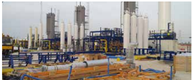
Assembly of the plant at site
