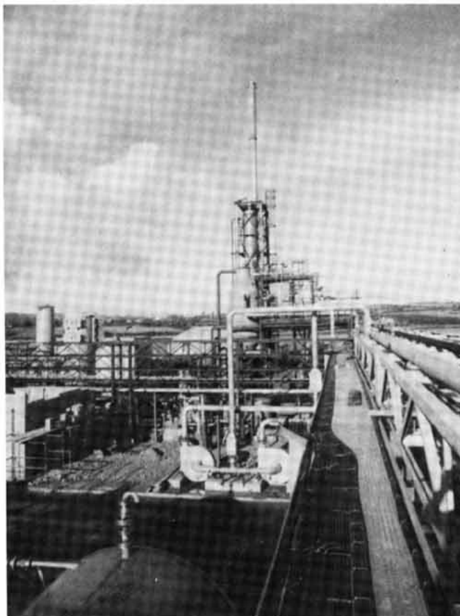
Fig. 3: Incinerator for the simultaneous combustion of chlorinated hydrocarbons and organically loaded brine.
