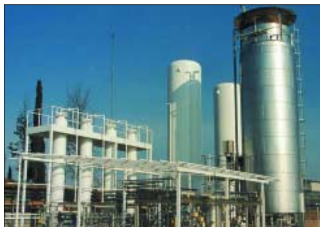
Fig. 5. Methanol cracker with PSA.
