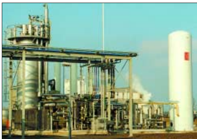
Fig. 3. Steam reformer with PSA.
