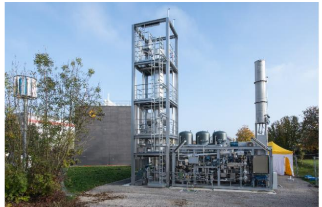
Fig. 2: Biological methanation plant ©RES
