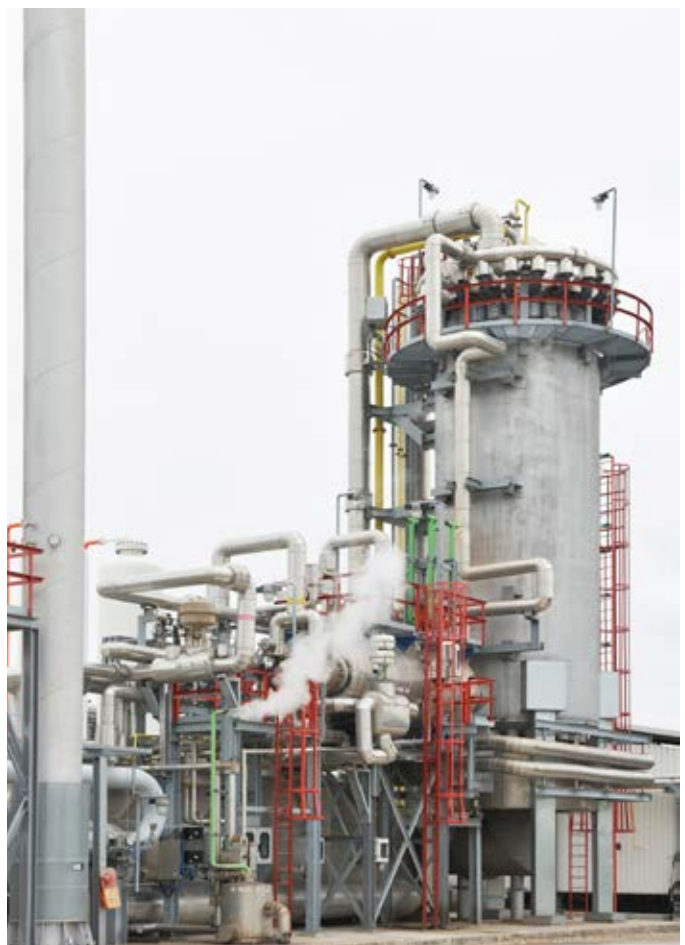
Steam reformer for 4000 Nm 3 /h hydrogen (purity 99,9%)
