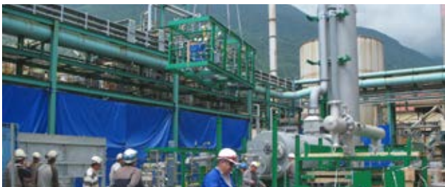
Placement of skid on prepared foundation
