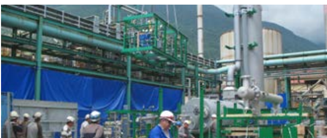
Placement of skid on prepared foundation
