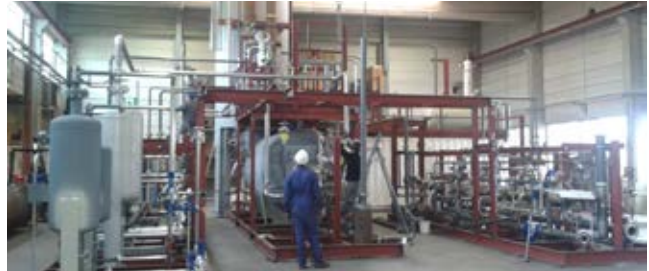
Pre-assembly of the plant in CALORIC's production facility
