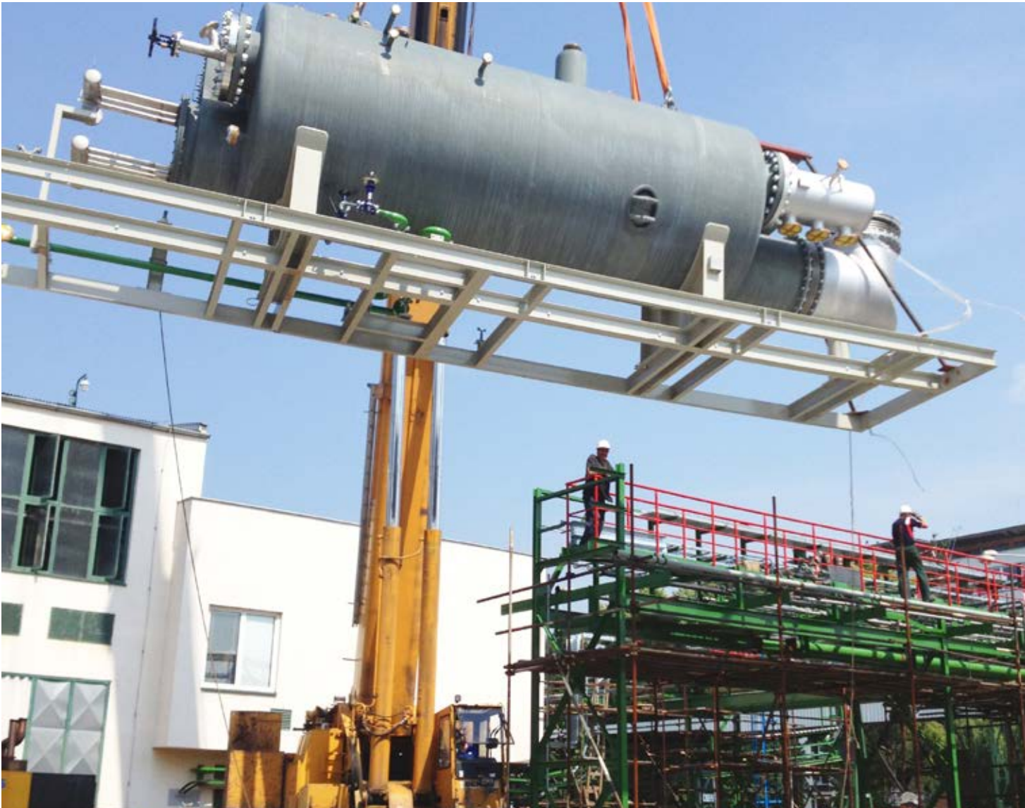
Skid mounted steam boiler is placed on prepared foundation
