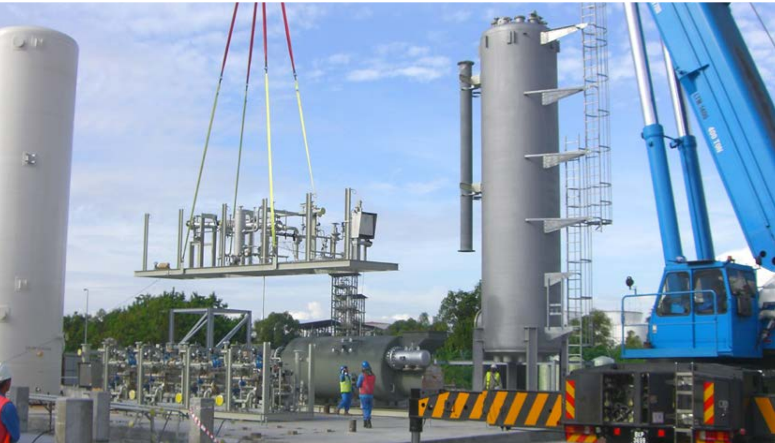
Natural gas steam reformer capacity 1750 Nm 3 /h during erection
