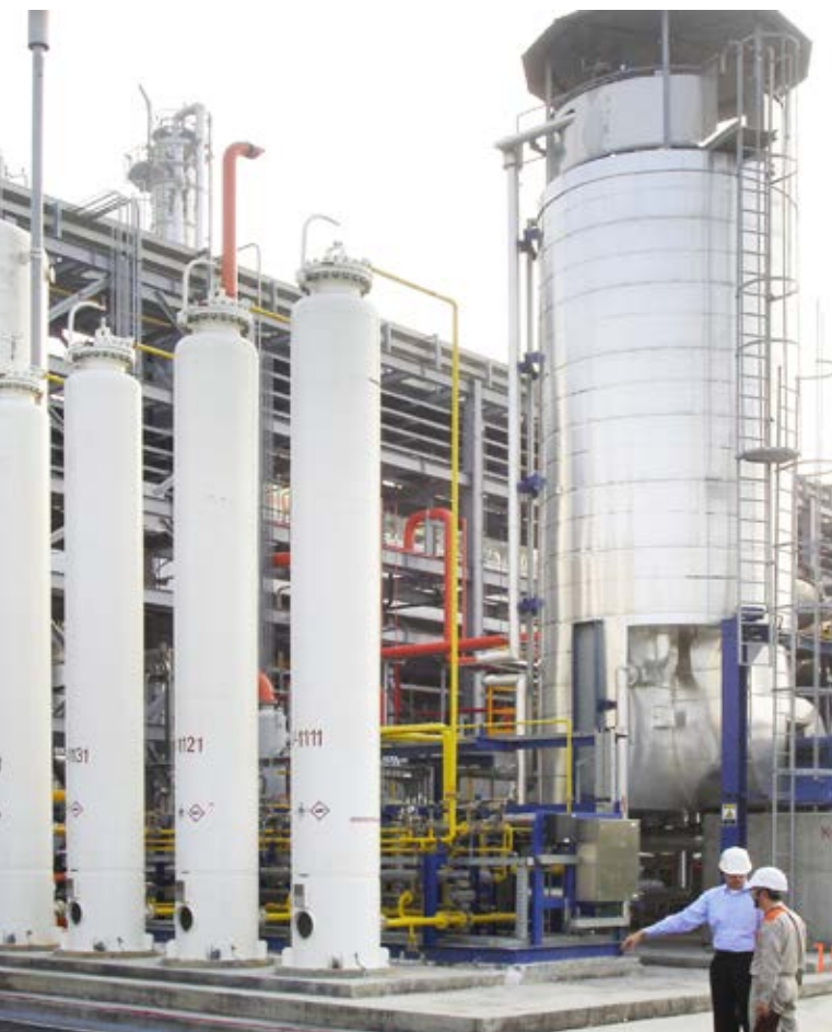
Methanol reformer for 840 Nm 3 /h hydrogen purity (99.9999%)
