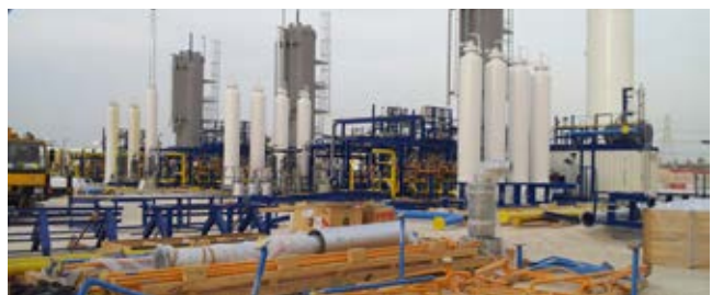
Assembly of the plant at site
